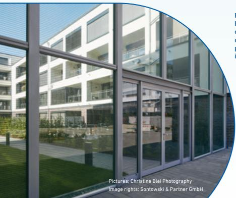
For a residential development surrounded by noise from three sides, 214 floor-toceiling HAFENCITY windows were used in order to reduce the external noise level at partially open windows from 66 dB to 30 dB indoor noise level.
